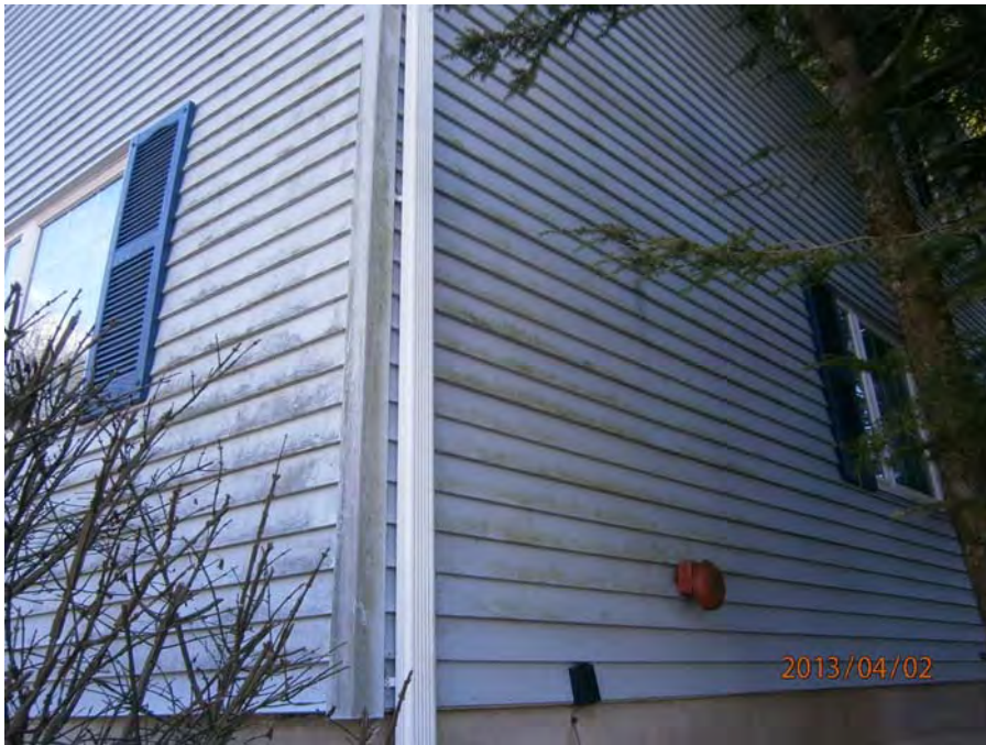
9. Vinyl siding - needs pressure washing
