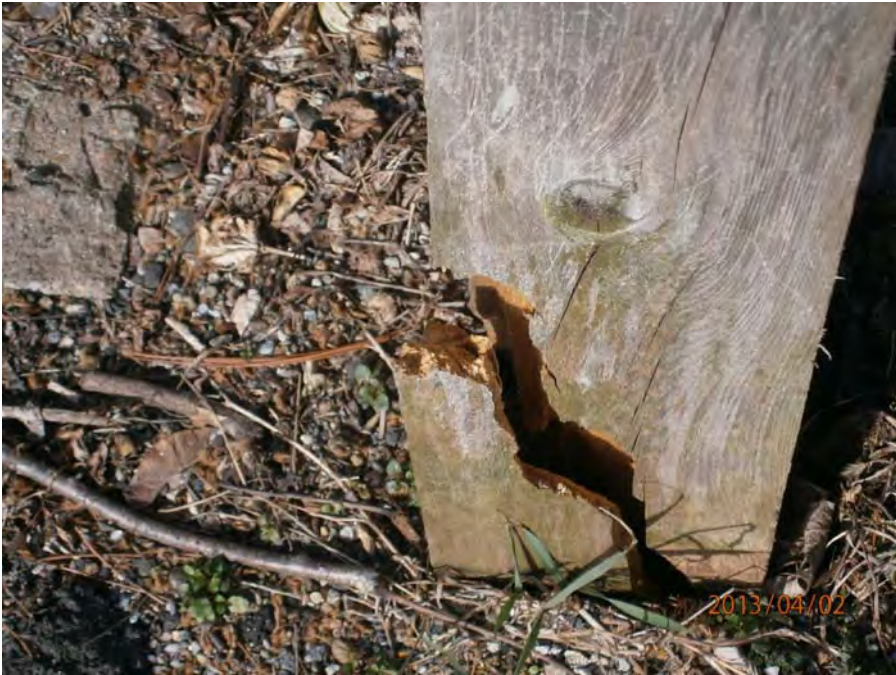
5. Dumpster enclosure support column damaged
