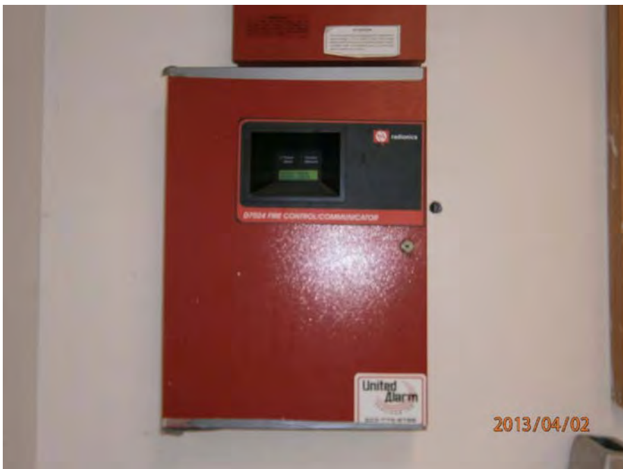
27. Zoned fire control panel
