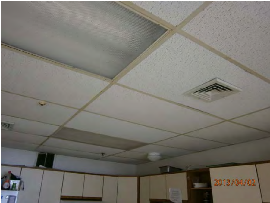
17. Typical suspended ceiling
