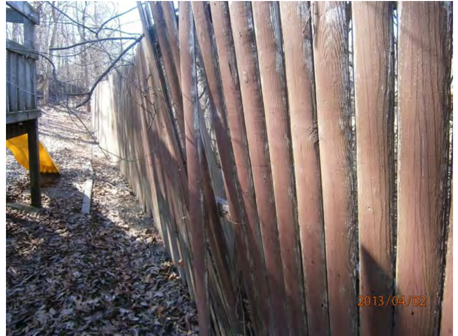
6. Wood stockade fence damaged
